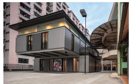
Completion of renovation in September 2022
