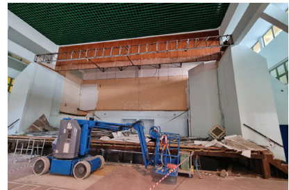
Multi-purpose hall (MPH) during renovation
