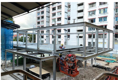
Construction of The Pods
