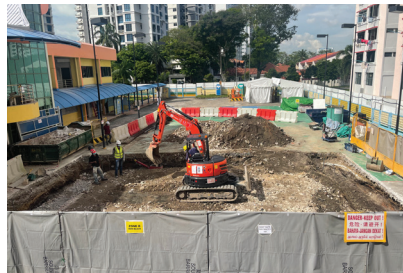
Renovation started in September 2021
